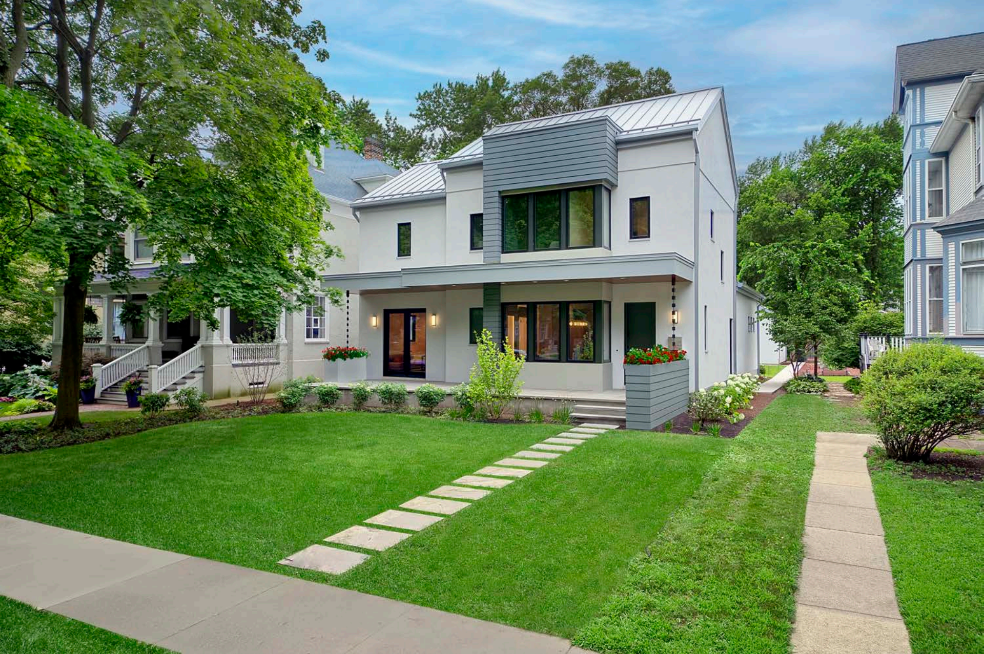
This home's modern, cantilevered porch overhang aligns with the heights of the neighbors' porches. Rain chains direct water from this overhang down into flower planters to divert water away from the home. The stucco and siding used on the front facade draw from the neighbors' material palette.
