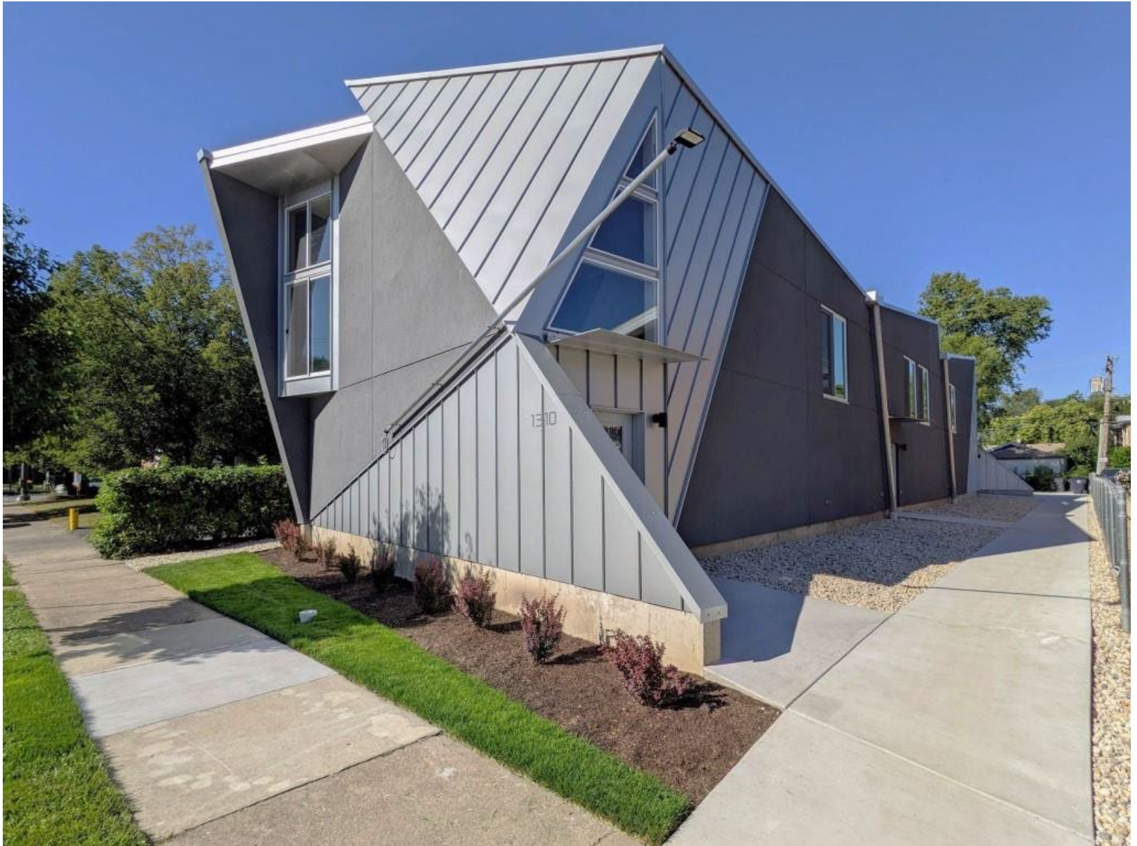
East facade facing Hartrey Avenue. Note the use of sustainable and energy efficient materials including continuous insulation and aluminum cladding, soffit and fascia.
