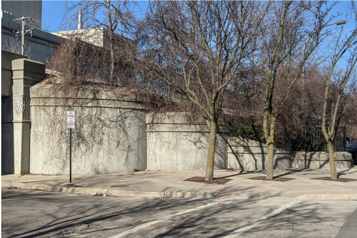
Abutment planters at Clark Street underpass. Credit: Tom Hofmaier
