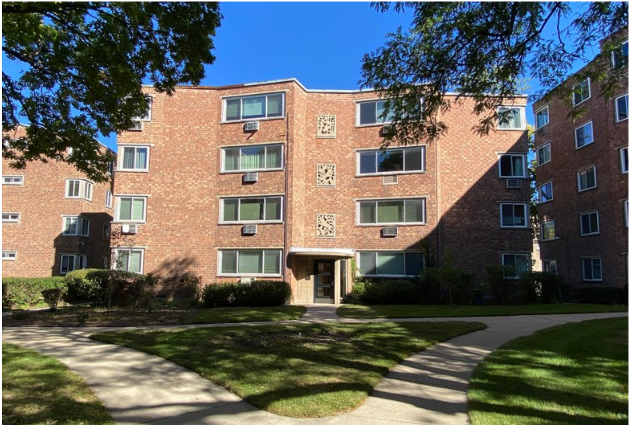
A view of 6155 N. Wolcott Ave. in Granville Terrace. Note the decorative cast concrete ornaments, identical to those used on the Sherman Gardens buildings in Evanston. Credit: Jack Weiss
