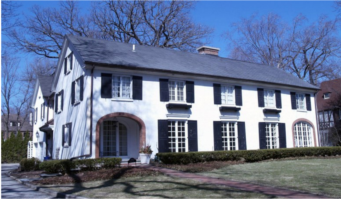
Rapp House, 2733 Colfax St., local landmark. Architect: Robert Seyfarth. 1916. Credit: The Lakota Group
