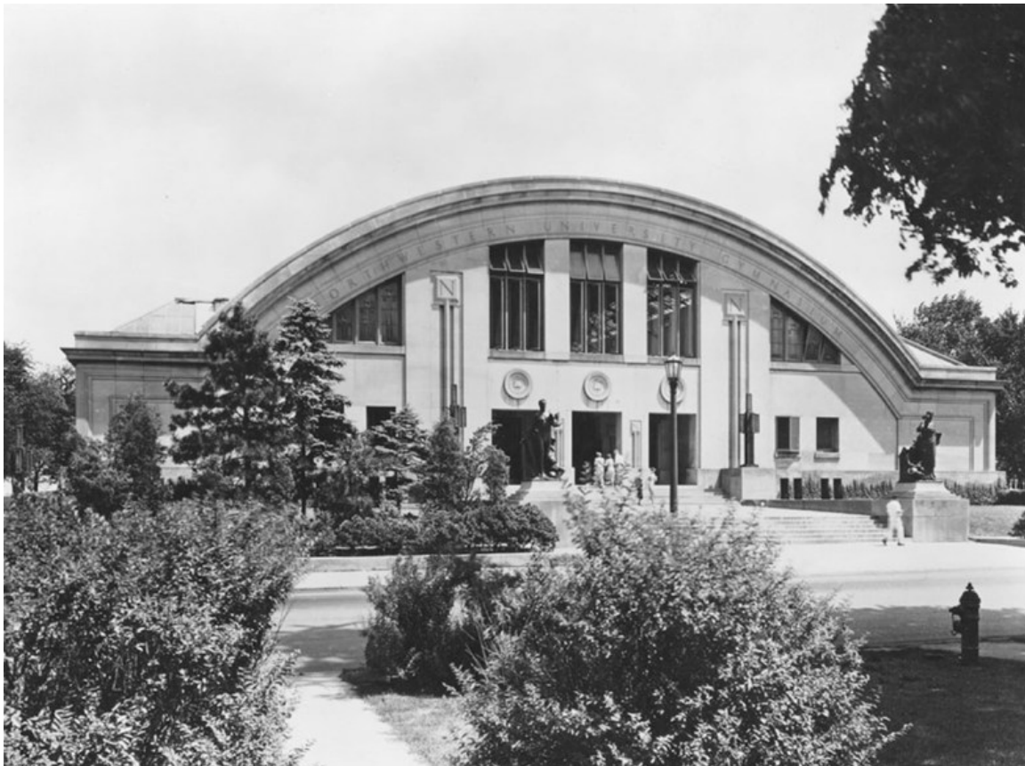
Patten Gymnasium, 2145 Sheridan Road. (Photo: University Archives, Northwestern Architecture)
